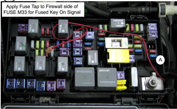
The RED wire is the one tied to the Fuse shown in the image above. This is the link that powers everything up. This is installed on the FUSED side of the fuse, the firewall side as noted in the picture. Be sure to clearance a bit of the fuse box to allow the RED wire not to be pinched when the fuse box is put back together, this is at the locations identified by the A in the image above.
